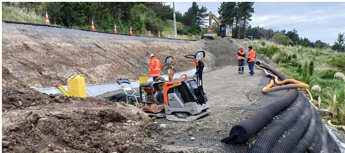
Figure 5: Emergency works in Taranua following Cyclone Gabrielle.
